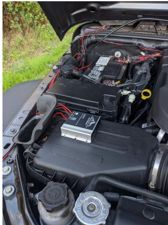
*Above is the charge controller mounted on the air intake box of a Jeep Wrangler JK .
